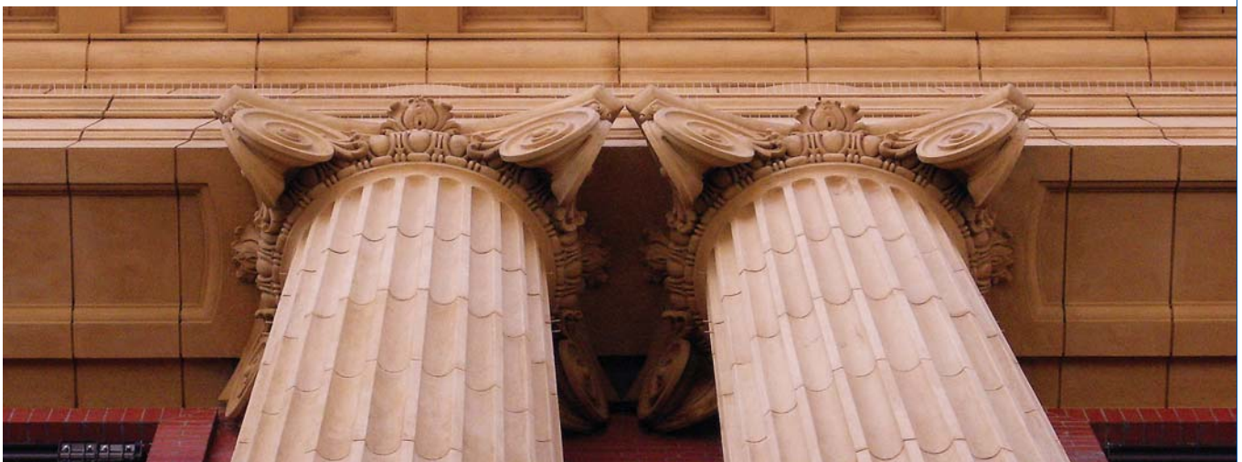
Old Mail Exchange Restoration Melbourne CBD.
